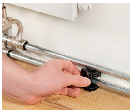
1. Attach lower part of mounting bracket rotated around 180°
