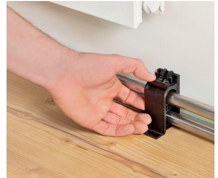
3. Attach upper part and tighten spring claw
