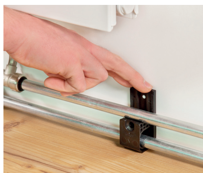
2. Insert wall holder plate and screw in place
