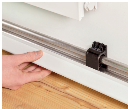
5. Swivel baseboard upwards
