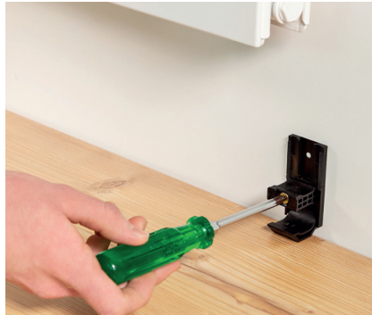
1. Attach wall holder plate and lower part of mounting bracket
