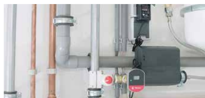
The Flexcon PA AutoFill monitors the pressure in the central heating system. With a permanent connection to the water pipe, the system is automatically topped up to the required pressure level whenever it drops.
