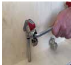
The KFE allows for fixing with an allen key, preventing damaging the outside.
